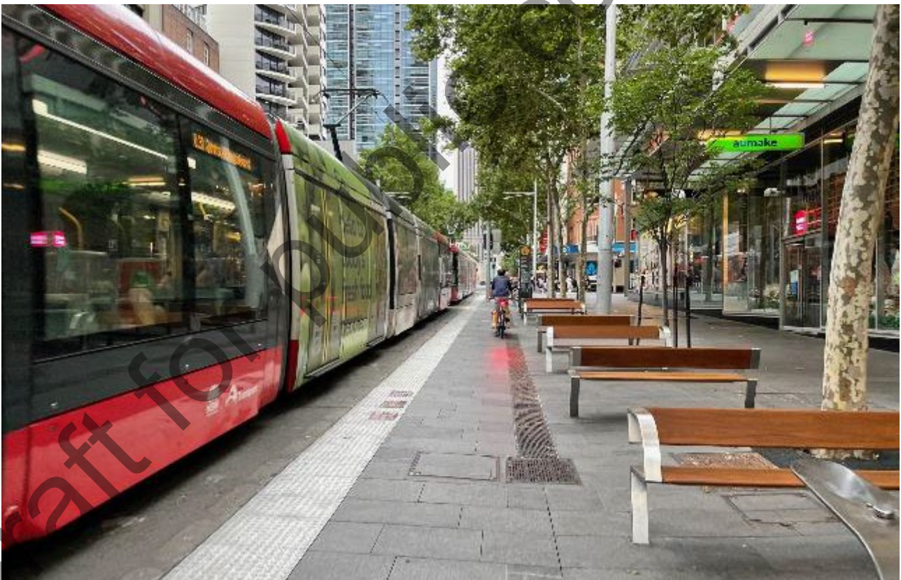
Figure 1-1 George St, Sydney, NSW Light Rail with outdoor seating and space
