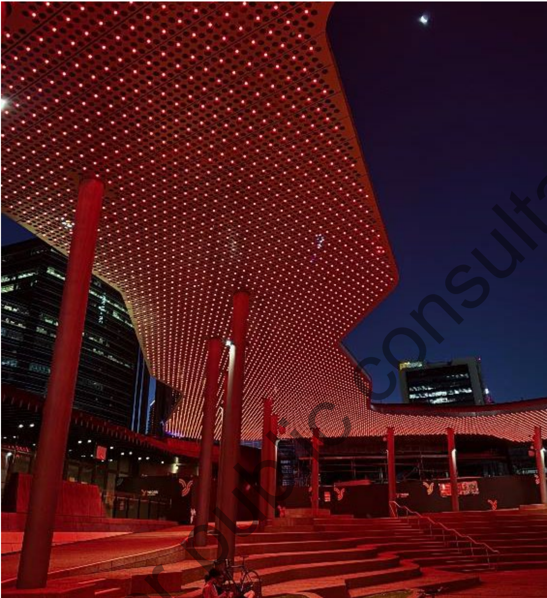
Figure 7-1 Karak Walk at Yagan Square in Perth, where the train line was sunk underground to create a large public space above ground, adjacent to Perth's central train and bus station
